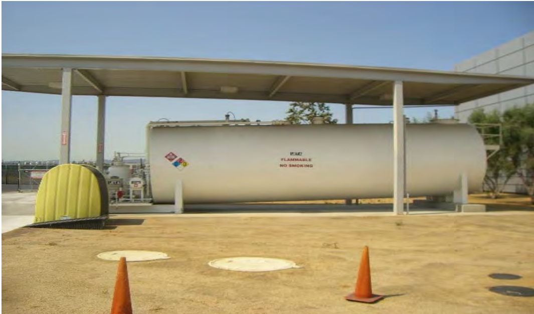
AVBASE ABOVE GROUND FUEL STORAGE TANK
