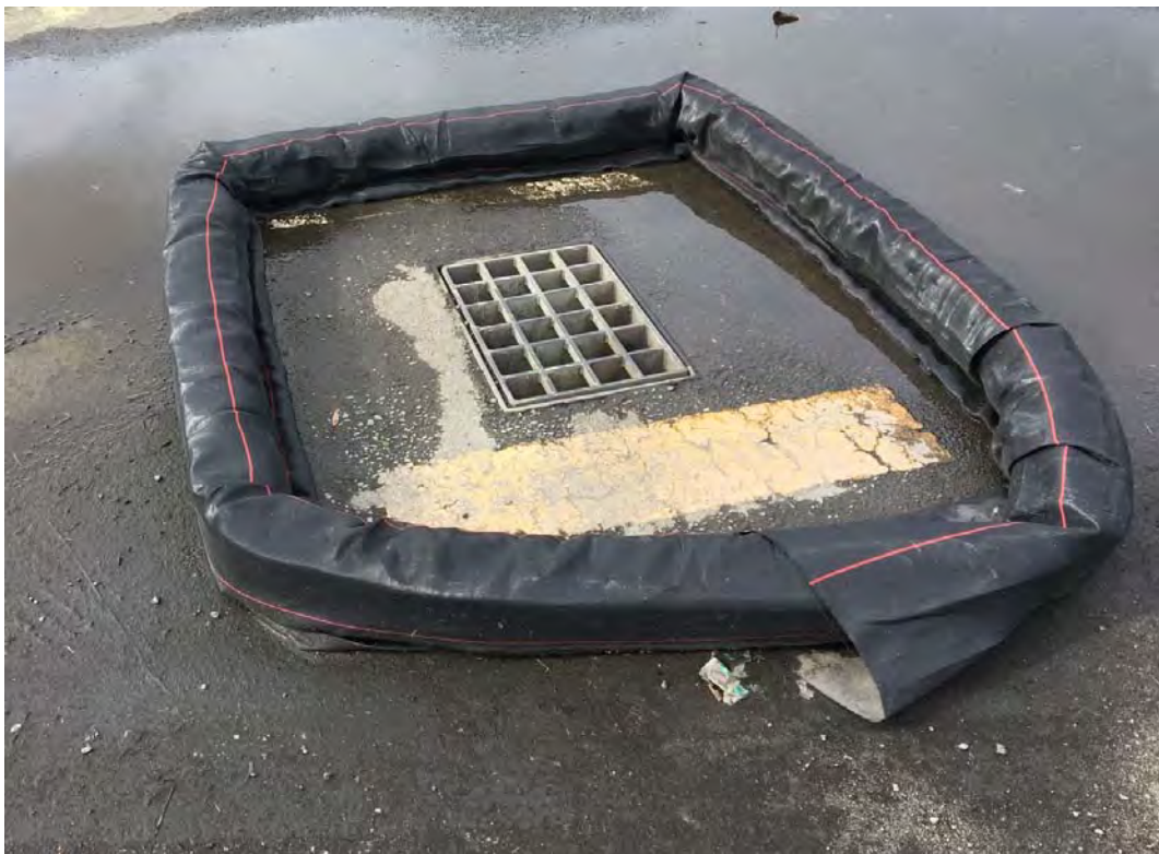
INLET PROTECTION AT SOUTH MAINTENANCE YARD
