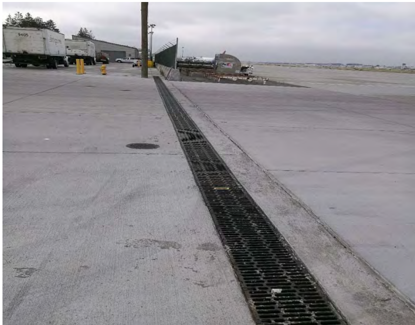
TRENCH DRAIN AT NORTHEAST PARCEL STORAGE AREA
