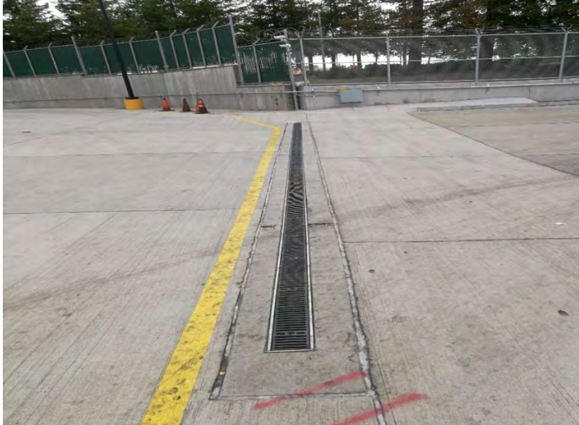
TRENCH DRAIN AT NORTHEAST PARCEL STORAGE AREA
