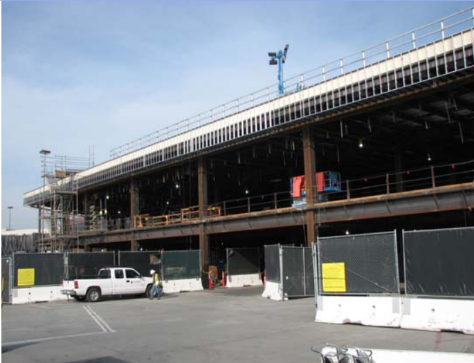
Bump Out Steel Completed
