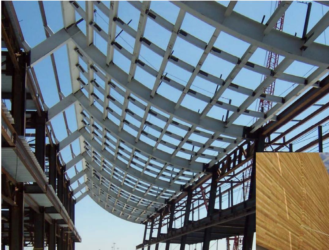
North Concourse Structural Steel
