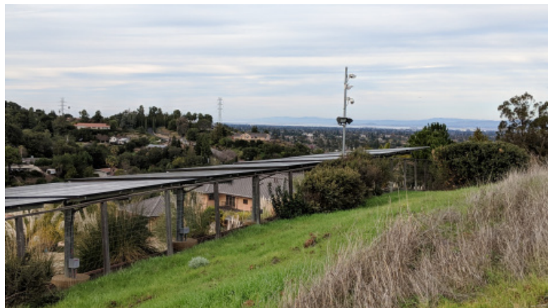
Example of solar panels on/next to a fence
